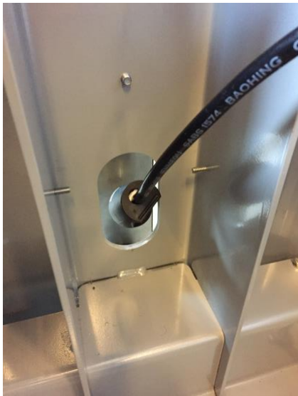
View from inside the cabinet.
