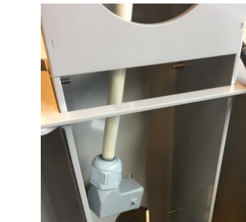
View from inside the cabinet.
